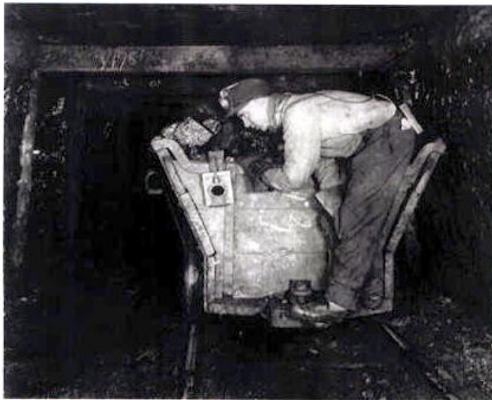
Figure (3) a coal miner standing on the back of a car in a mine tunnel in the early 1900s. Notice that the sides of the tunnel are shored up with timber
