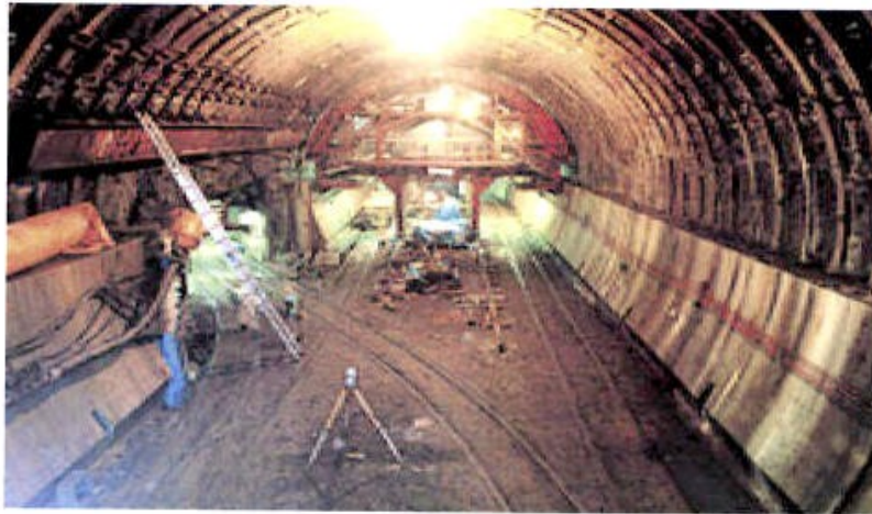
Figure (5) Construction of the Seikan Tunnel involved a 24-year struggle to overcome challenges posed by soft rock under the sea
